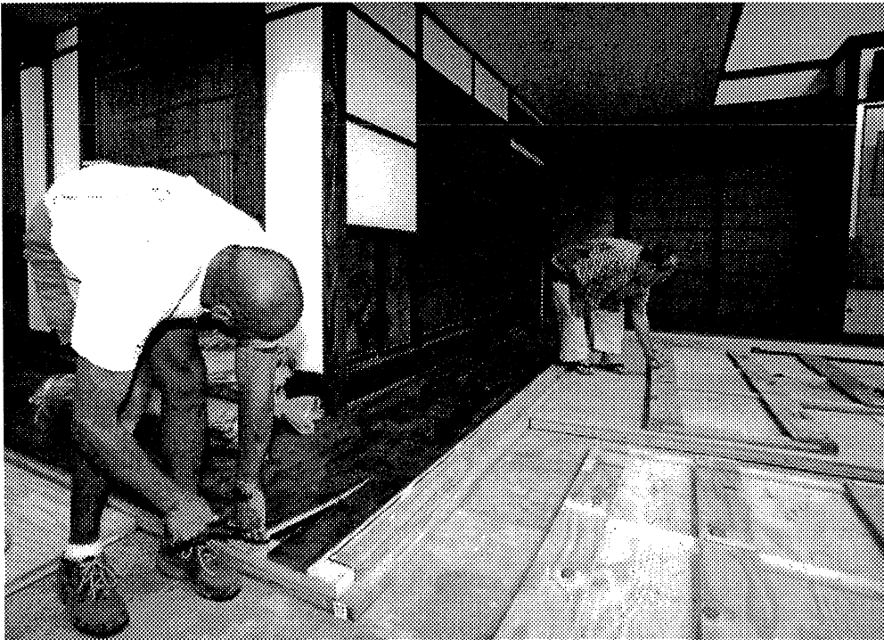
Sensei helping too? Daniel, our next door neighbor, working hard to finish over the weekend.
